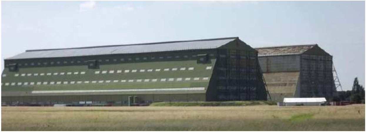
The colossal airship sheds at Cardington, Bedfordshire, which housed the R101.
