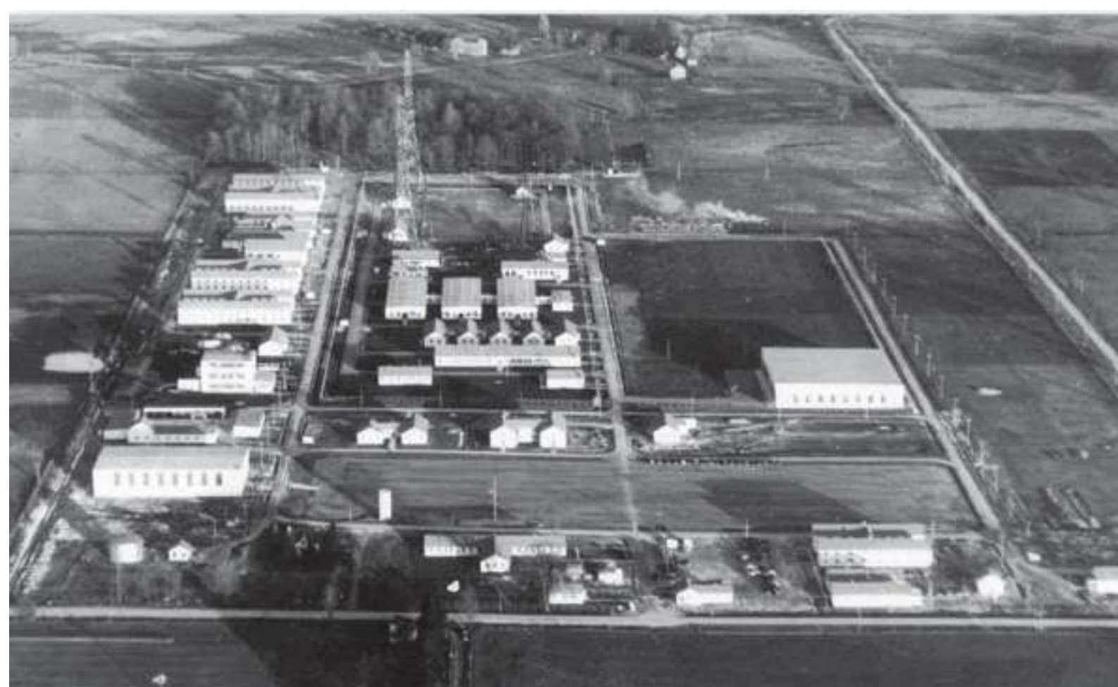
One of the most vital aids to the pilots of RAF Fighter Command in the defence of Britain was RDF, or Radio Direction Finding. Set up in a defensive perimeter codenamed 'Chain
