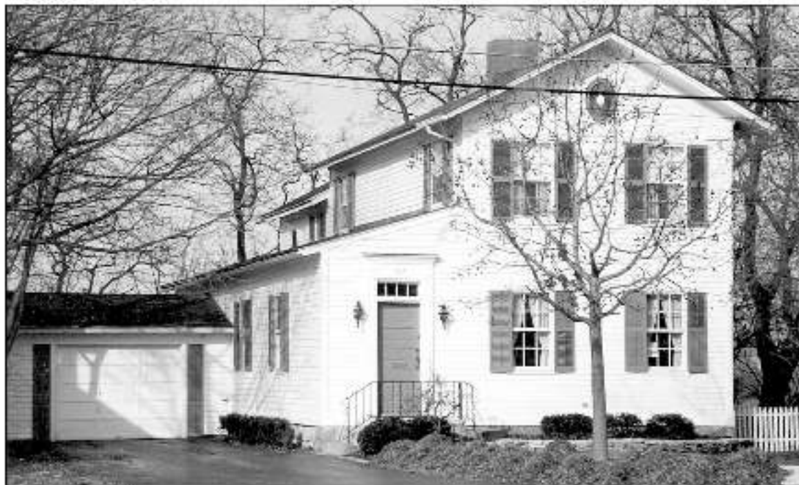
B. F. HOLLISTER HOUSE AT 407 WEST FRONT (BUILT IN 1830s). Benjamin Hollister, from Massachusetts, built this house whose roofline and elliptical fanlight in the gable reflect the earlier Federal period. It has a framework of hand-hewn timbers secured by mortise and tenon joints and wide-plank pine floors laid directly over logs. Hollister (brother of John, see page 12) ran a general store and was in the fur trade with the American Indians. He escorted parts of the Ottawa and Miami tribes to their exile in the west.
