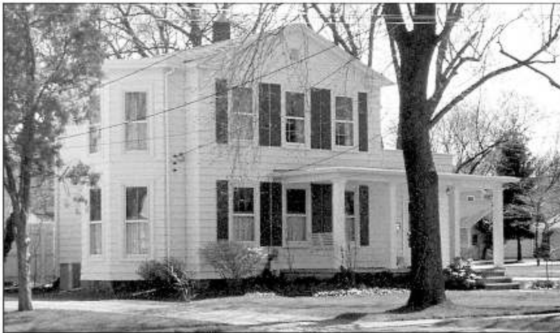
WAY HOUSE AT 529 HICKORY (BUILT IN 1830s). Believed to be built by a John Chambers, this house was the Willard V. Way family house for many years, and it once stood on the corner of Indian and Walnut where the fire department is now. Way came here from New York state and was a prominent lawyer, county prosecutor, mayor, and civic leader, but was considered by some to be rather miserly by nature. Upon his death, they were surprised to learn that he left the village money to build a library and to buy books, six lots for a park, his house, and funds for a school scholarship. The house was moved in the early 1900s.
