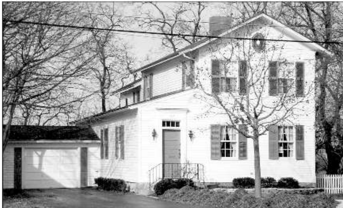
B. F. HOLLISTER HOUSE AT 407 WEST FRONT (BUILT IN 1830s). Benjamin Hollister, from Massachusetts, built this house whose roofline and elliptical fanlight in the gable reflect the earlier Federal period. It has a framework of hand-hewn timbers secured by mortise and tenon joints and wide-plank pine floors laid directly over logs. Hollister (brother of John, see page 12) ran a general store and was in the fur trade with the American Indians. He escorted parts of the Ottawa and Miami tribes to their exile in the west.
