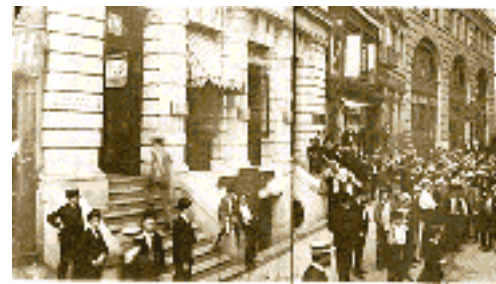
Wall Street's curb market, 1902 Courtesy, Library of Congress
