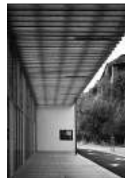
Primary school extension, Saillon
