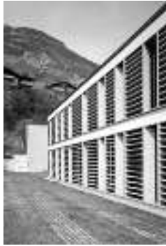
Primary school extension, Saillon
