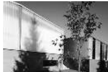
Gymnasium and multi-use hall, Renens
