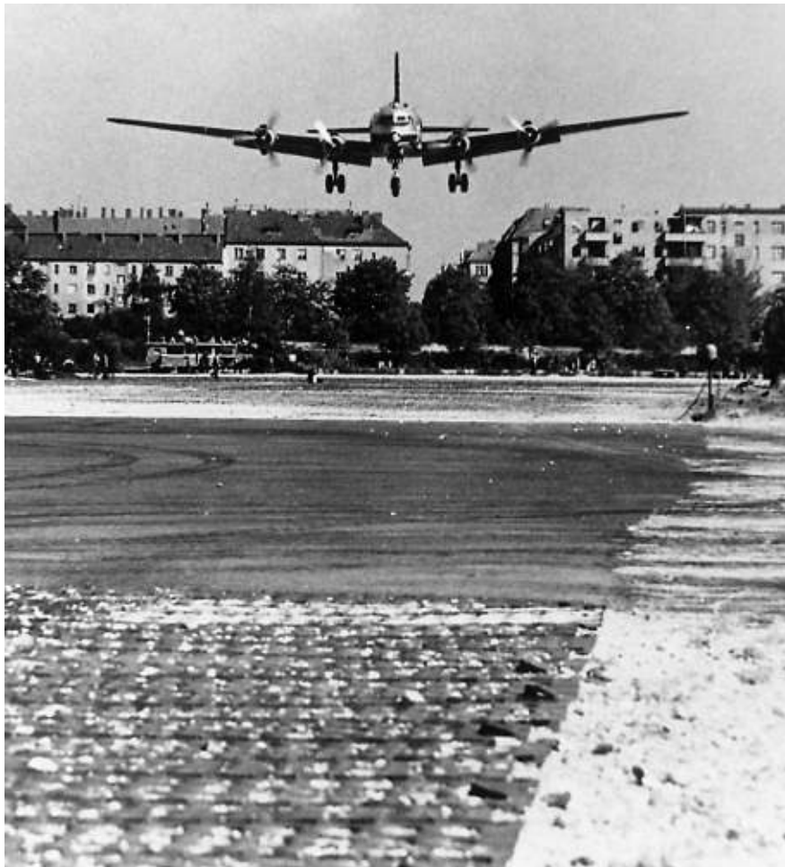
A C-54 comes in over apartment buildings to land at Tempelhof. The runway was covered with temporary pierced-steel planking (visible in foreground) that made for a noisy, bone-jarring landing. The planking was later replaced with pavement.
